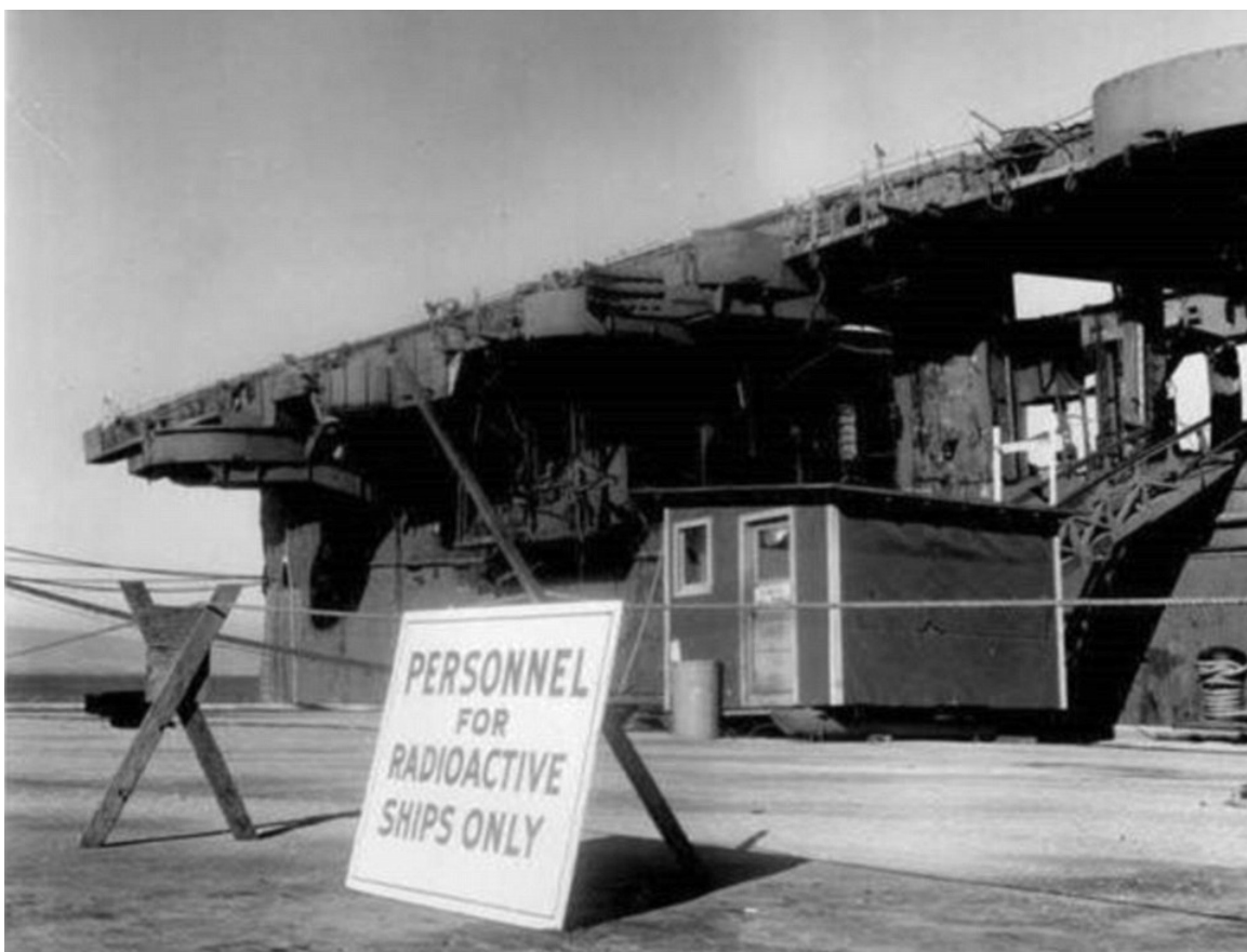
Figure 9 - A sign in front of the Ex-USS Independence anchored at HPS, reading "Personnel for Radioactive Ships Only" (NARA)
