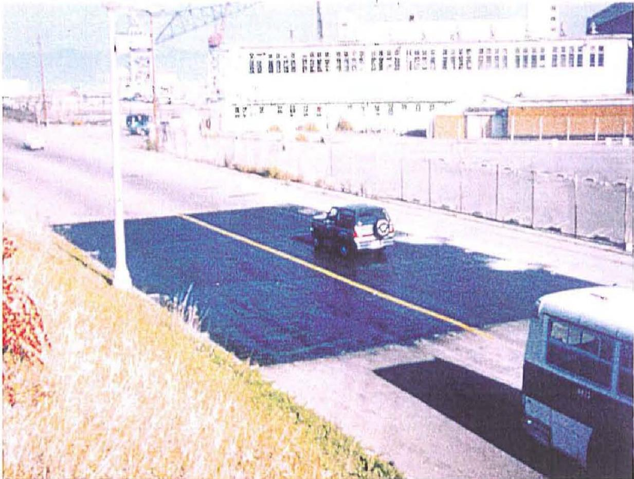
Asphalt at HPNS made out of HPNS sandblast grit
